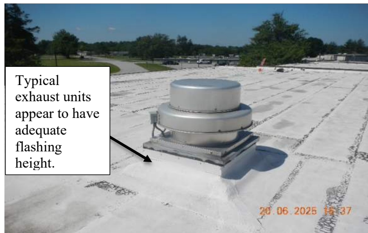
Photo 10 – Typical flashing at exhaust unit on upper roof.
