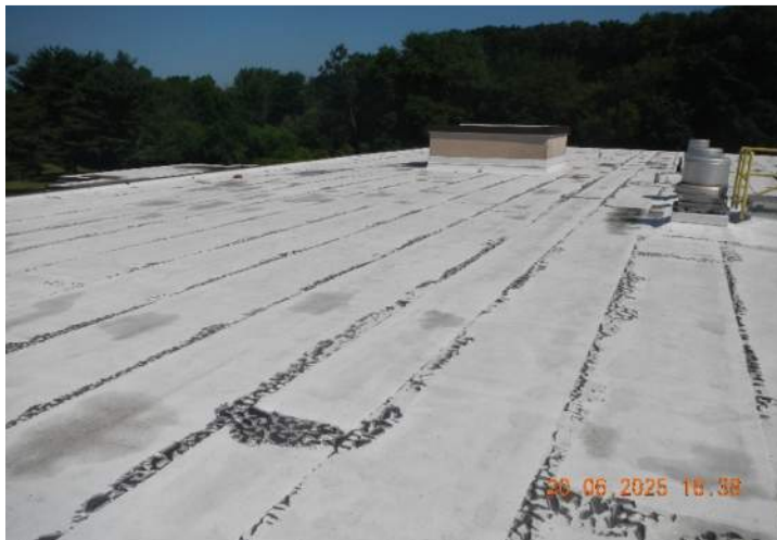
Photo 2 – Overview of upper roof section and small penthouse roof.
